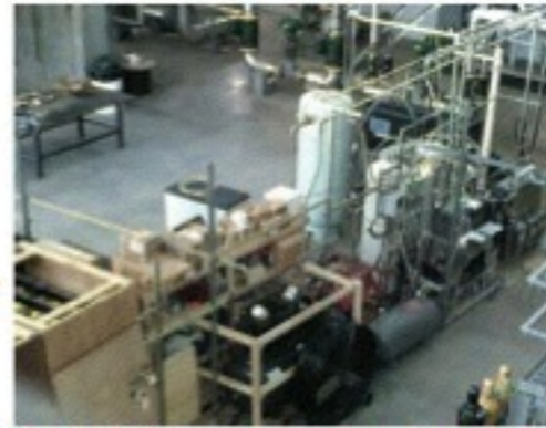
DarkSide's argon separation plant at Kinder Morgan Doe Canyon CO 2 facility
