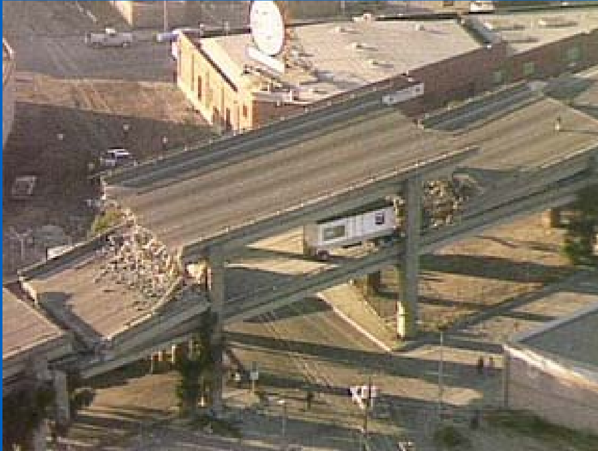
Loma Prieta, CA 1989
